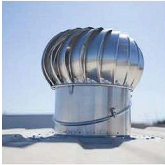
Roof Top Turbine FIG 1.1
