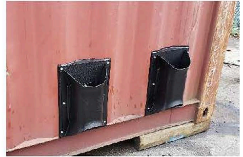
Floor Level Fume Extraction FIG 1.3
