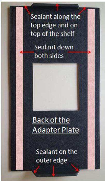
Use a good exterior sealant such as Sikaflex, as per the drawing on the left. Ensure to load up the top shelf on the plate (fits under the upper structural cross bar of the container), as seen below. Sealant down the side flanges and the bottom profile (that keeps the low pressure inside the system)
