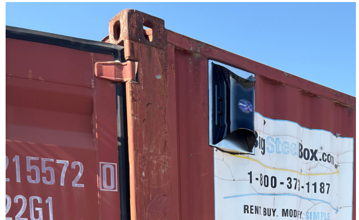
An Exhaust installed on a side wall
